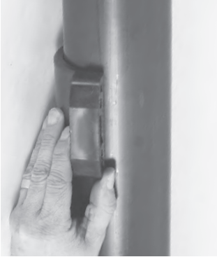
1. Position lower half of saddle around pipe.
