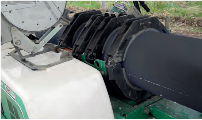
Butt Fusion machine prior to commencement of fusion process
